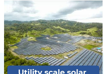
Utility scale solar
