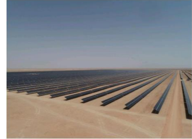
Oman 125MW Solar Project
