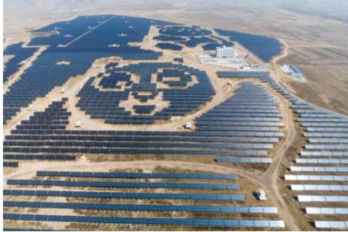
'Panda' Power plant-29.21 MW
